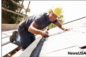
A new roof is the ultimate “curb appeal” enhancer.
